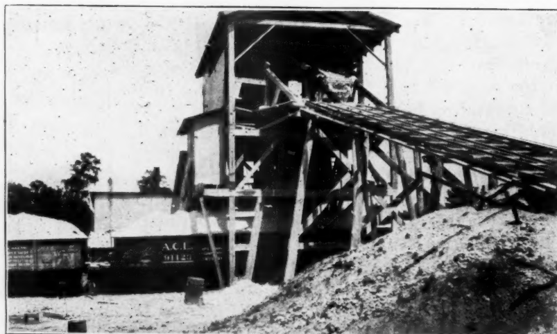
Loading Road Base Directly Into Cars
